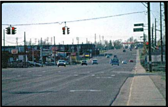
Figure 4: South Golden Road prior to reconstruction (5).
